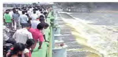
WATER GUSHES OUT OF THE KALLANAI DAM BUILT OVER THE CAUVERY IN TIRUCHI, TAMIL NADU
