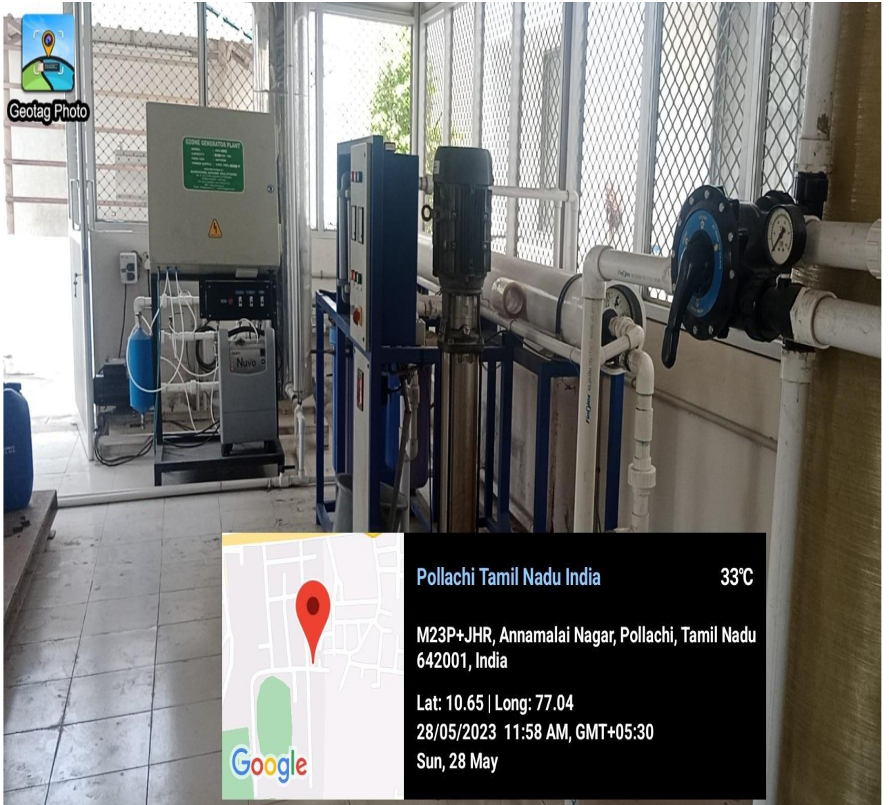
RO plant located inside the campus for filtering and desalinating the water
