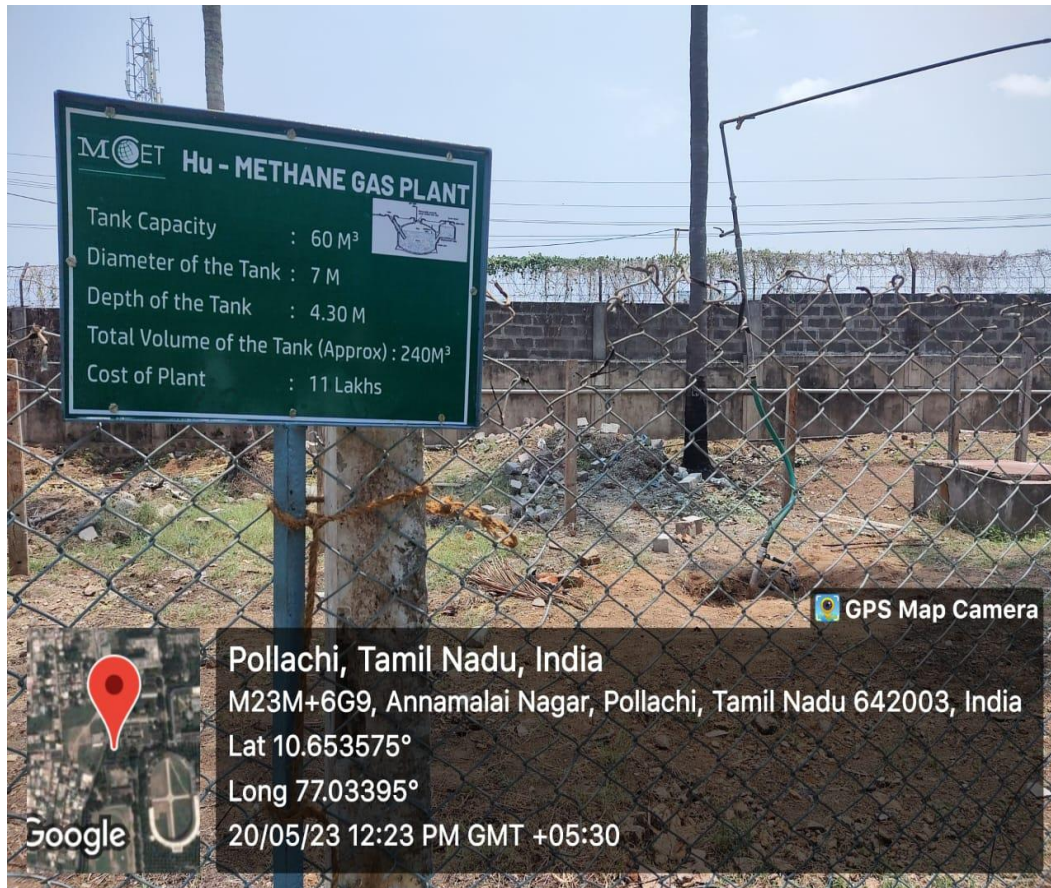
Fig.2.2 60 M 3 TANK CAPACITY BIOGAS PLANT
