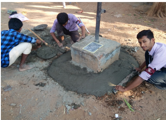
Cementing uneven surfaces
